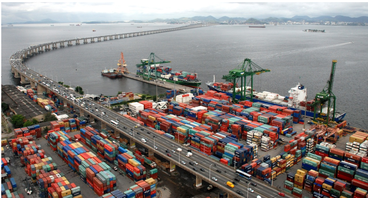
Figure 2. Storage area and port side view of Container Terminal of Rio de Janeiro, Brazil [19].
